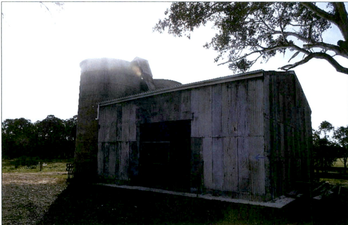
Photograph 13: Sheet metal barn and silos located 120 m northwest of the proposed solar array area
