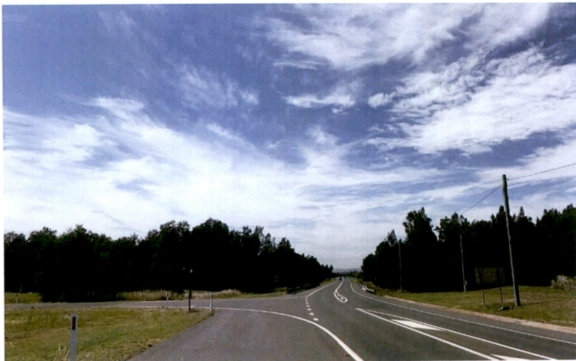
Photograph 10: Wine Country Drive, Wills Hill Road intersection showing line marking, passing and turning lanes
